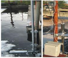
Control of the dissolved oxygen concentration in a wastewater treatment plant
